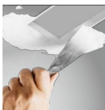
skimmed into plaster-board ceiling (trimless)
