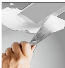
skimmed into plaster-board ceiling (trimless)
