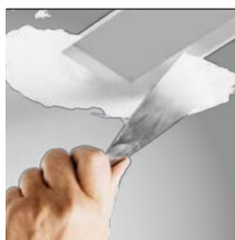
skimmed into plaster-board ceiling (trimless)
