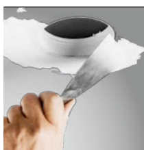
skimmed into plaster-board ceiling (trimless)
